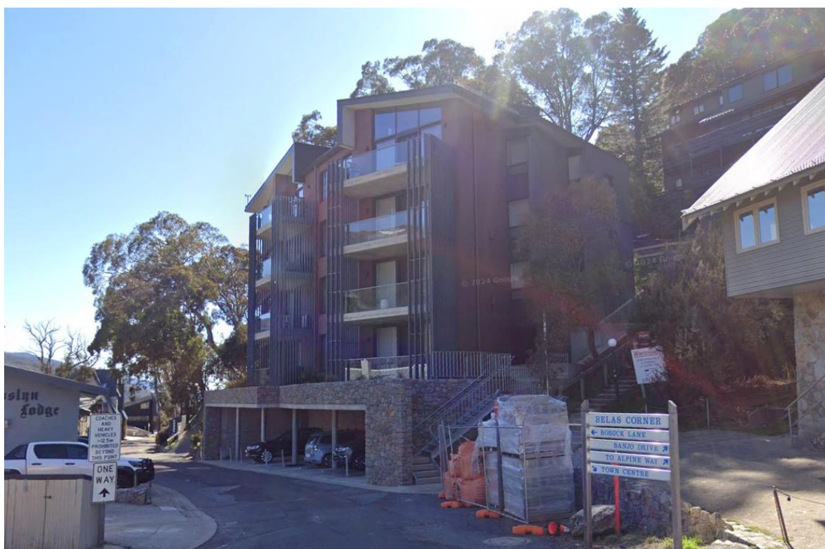
Figure 2 | The existing building on the site (source: Google Street View)
